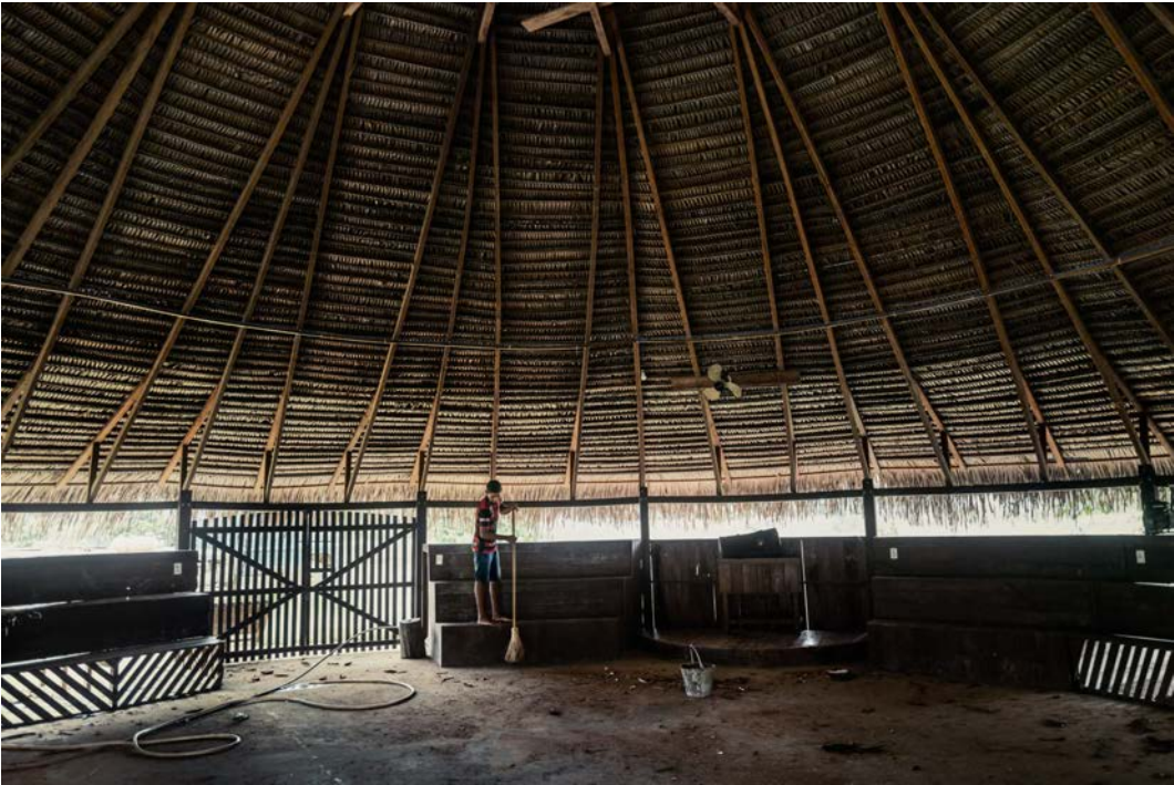
The Yorenka Tasorentsi health centre, opened by Benki Piyáko, is built according to the principles of traditional Asháninka architecture, which places great importance on the geometry of the roof
